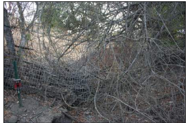
Figure 17: Fencing on south side of Bailey Bridge.
