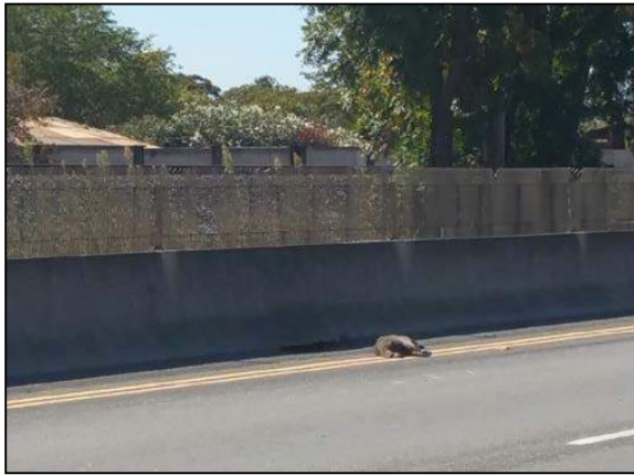
Figure 20: Monterey Road median barrier.
