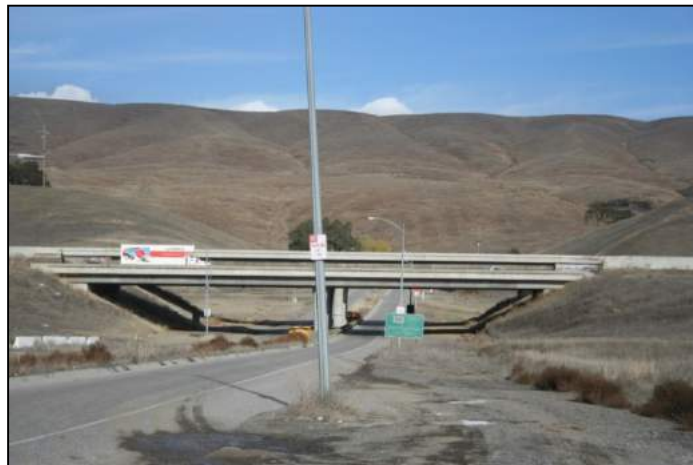
Figure 42: Highway 101 Golf Course Drive Underpass.
