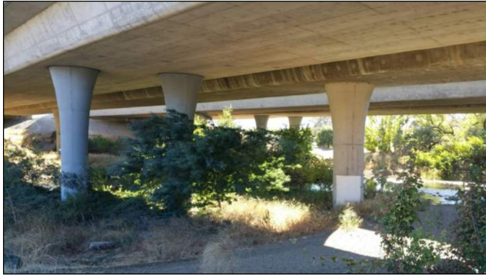
Figure 49: Highway 101 Coyote Creek Underpass.
